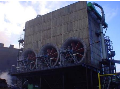
2.5MW air handling units
